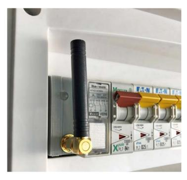
Place the transmitter preferably in a free position on the din rail. Only induction from the wires is sufficient for the actual power supply. The recovery occurs at approx. 3x5 A or 1x13 A. If the transmitting the antenna is shielded, e.g. by a metal cabinet or metal door, it is necessary to lead the antenna out of this shielding. A 50 ohm coaxial extension cable can be used, or a larger 886 MHz antenna with a longer feed cable.
