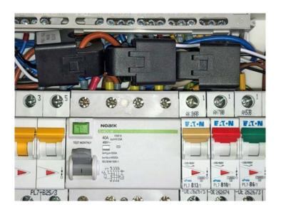
Install metering transformers in a location where the total consumption in the building can be measured. For example, at the supply to the house switchboard.
